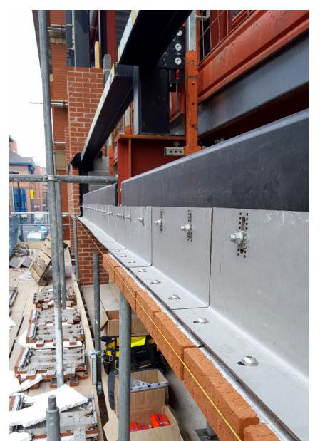
Lateral adjustments and gauging between coursing is achieved by sliding the unit left and right. The square nut allows the unlimited finite adjustments.
