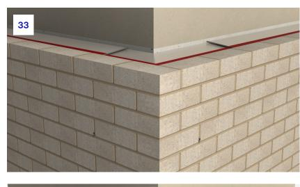
**33.** Brickwork can then continue up the façade ensuring that brick ties are installed as per the design team instructions.
