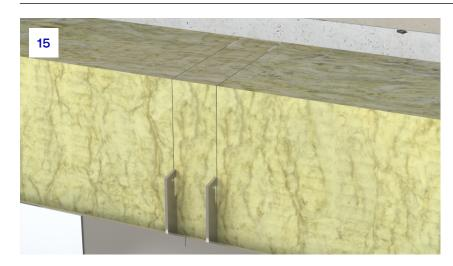
**15.** To the next side of the bracket, a piece of insulation should be installed again up to the bracket to ensure continuity.
